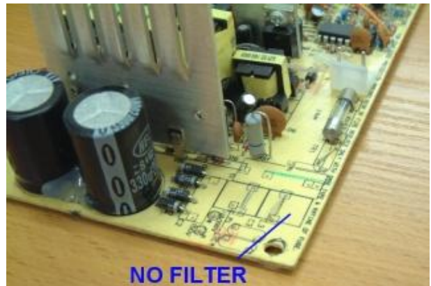
Not mounted filter components. Power supply manufacturer save on several dollars.
